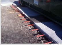
Concrete pavement replacement project at retail Distribution Center – Traditional reinforcement bar ("rebar") to provide load transfer to adjoining panels.
