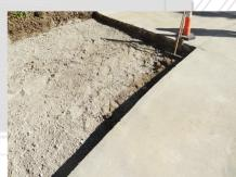
Concrete pavement replacement project for Municipal street repairs – Concrete panel removed and base rock being placed prior to dowel bar placement and compaction of base rock.
